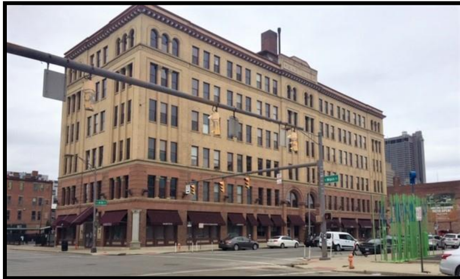
2020 Northwest Corner of Main and Fourth
