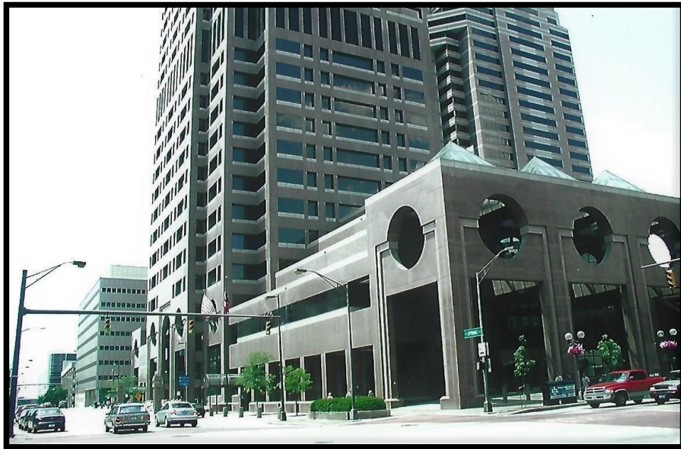
2005 Northwest Corner of Spring and High
