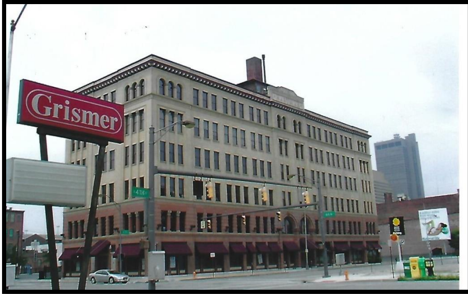
2005 Northwest Corner of Main and Fourth
