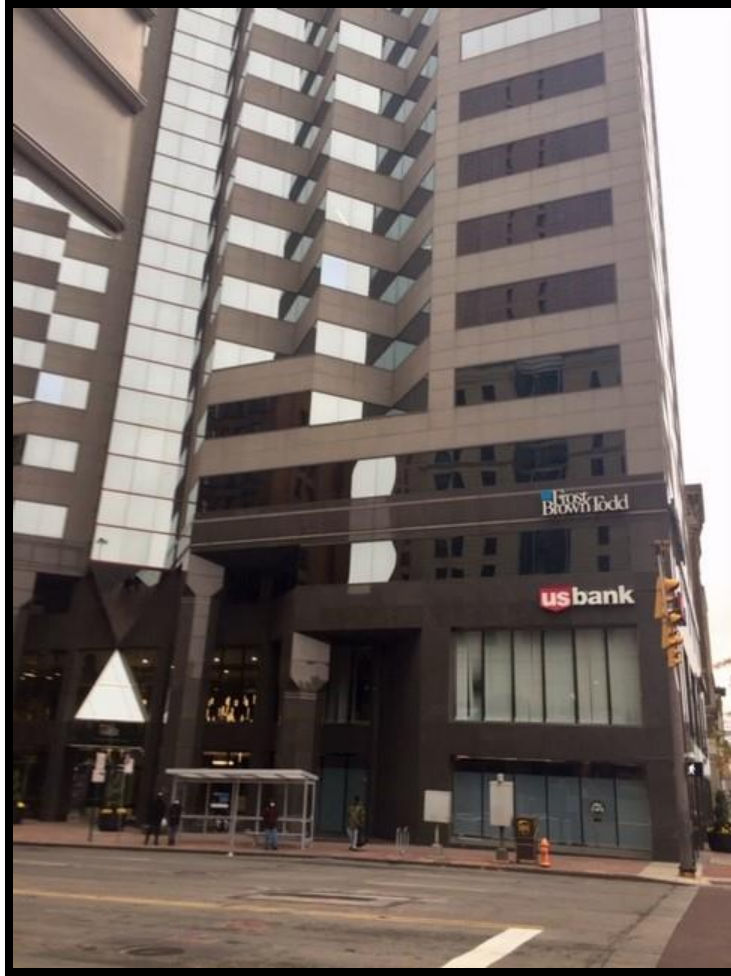
2020 Northwest Corner of Broad and High
