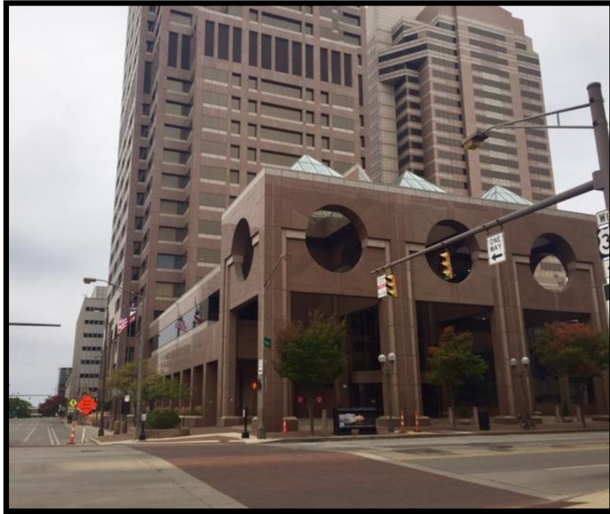
2020 Northwest Corner of Spring and High
