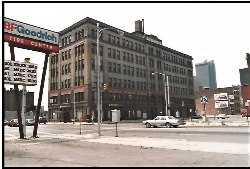
1985 Northwest Corner of Main and Fourth
